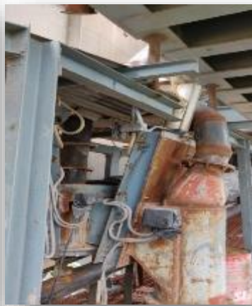
Preheater top feeding airslide modification
