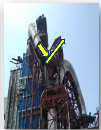
AQC : Booster Fan Bypassed Route After Modification
