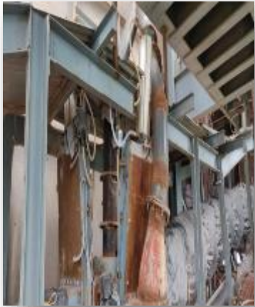
Preheater top feeding airslide modification
