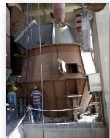
Cement Mill Classifier & CA Fan Upgradation
